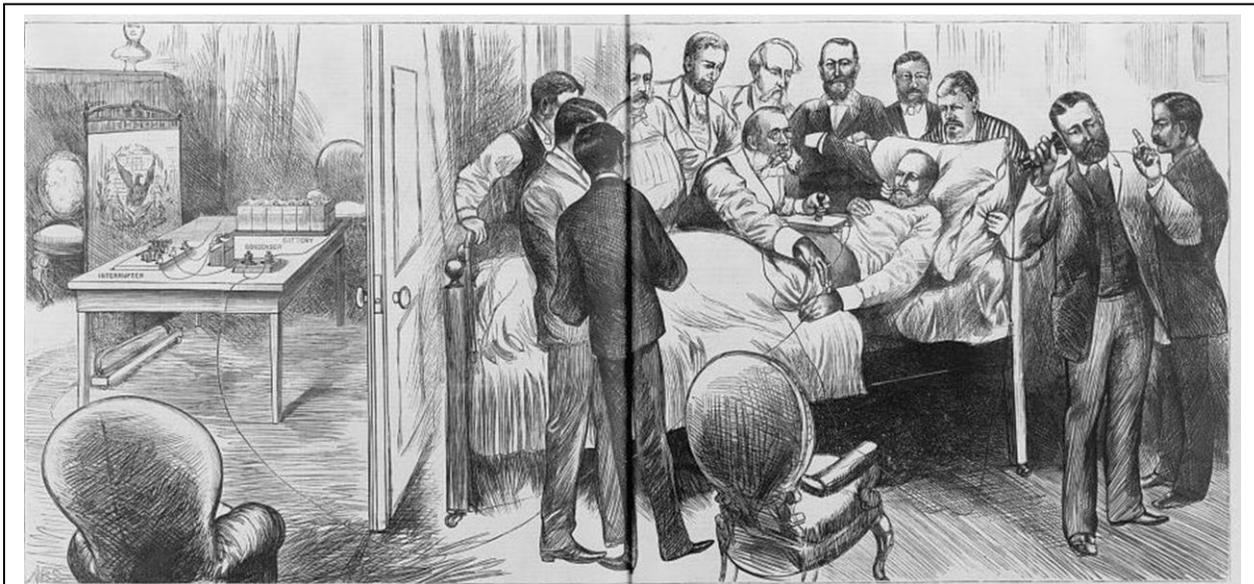
**Figure 3:** This drawing shows one of Bell's attempts to locate the bullet. The electromagnetic apparatus is located in the neighboring room on the left with wires running under the door. Bell is holding the telephone receiver on the far right while his assistant is moving a coil on the President's stomach. (Frank Leslie's Illustrated Newspaper, August 20, 1881, Downloaded From the Library of Congress)
